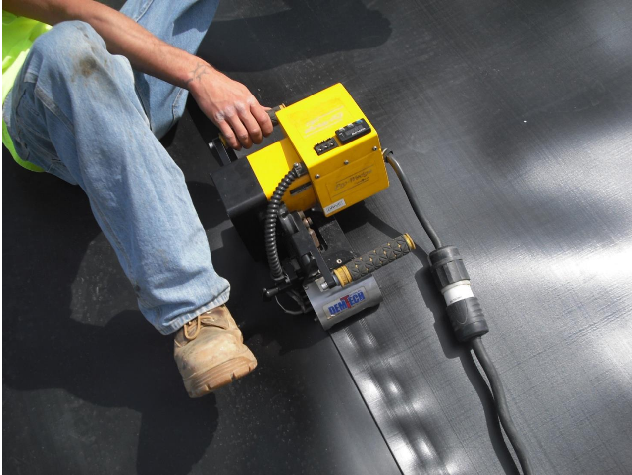
Dual track thermal fusion weld.
